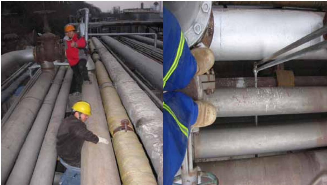
**Fig. 3. Example of Accessing a Difficult Tail Gas Analyzer Sample Point.**
